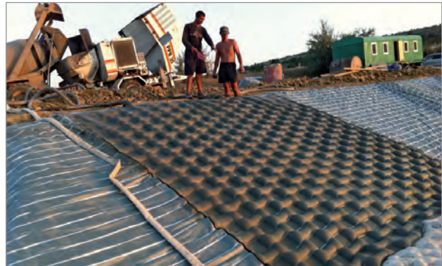
Installation of Incomat® Crib 10.100 at the upper slope
