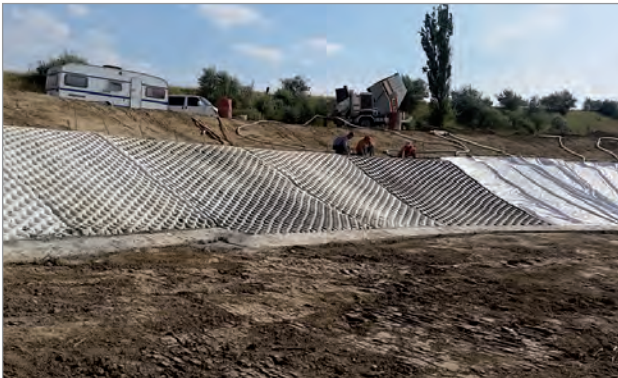
Installation of Incomat® Filterpoint C 60.148 at the lower part of the slope
